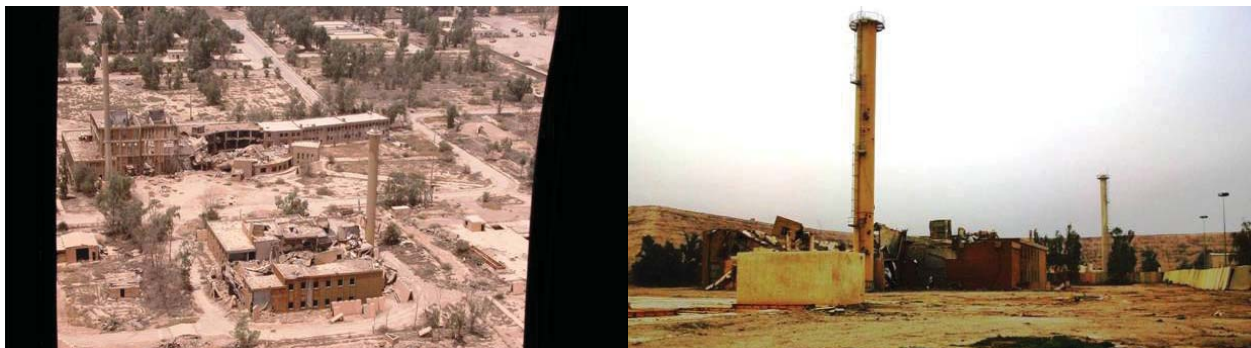
Left: View of an Iraqi nuclear facility from the air in 2005. Right: View from the ground in February 2009 after completing the first two phases of dismantlement.
