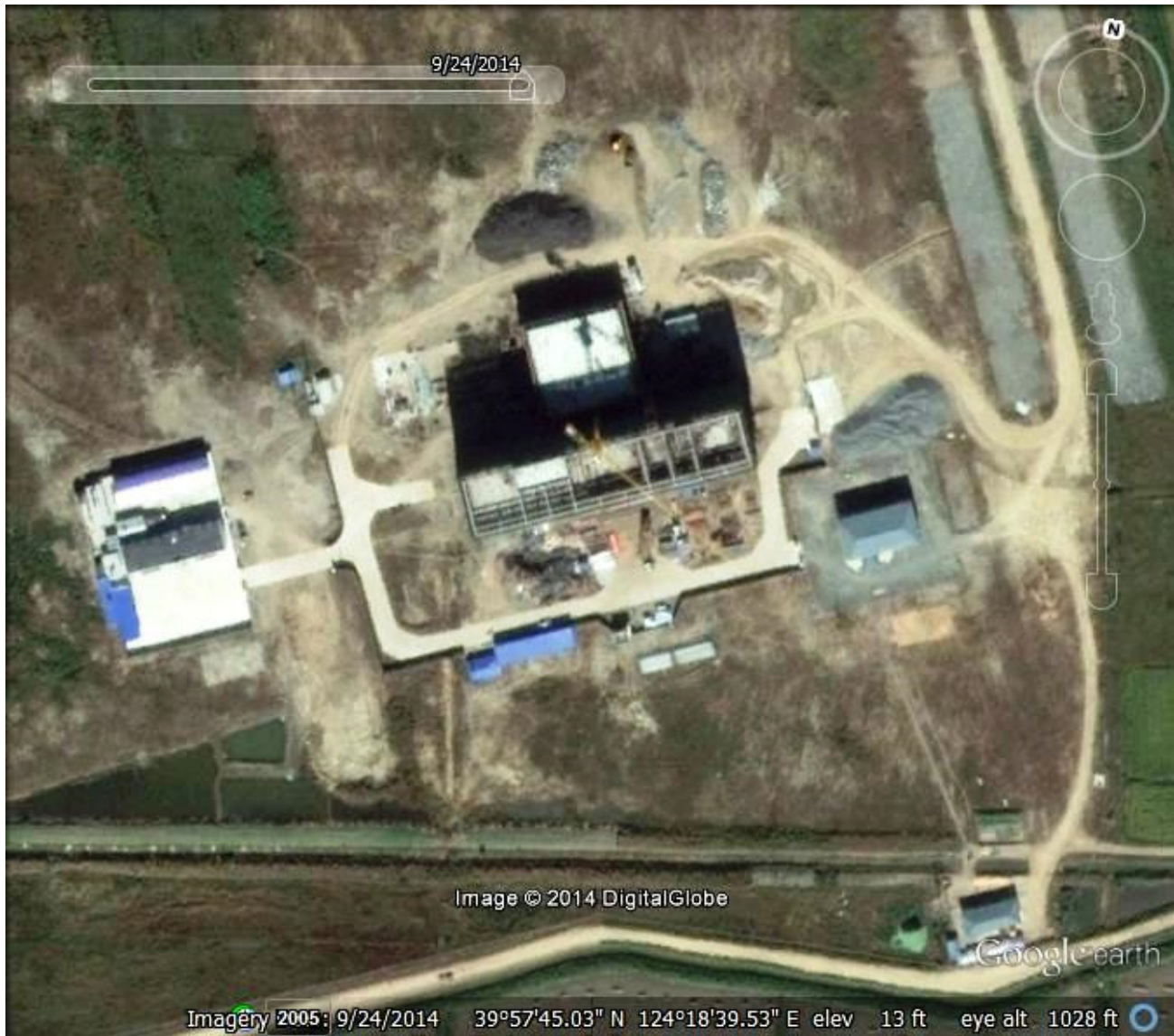
Figure 3. Building construction as of September 24, 2014.
