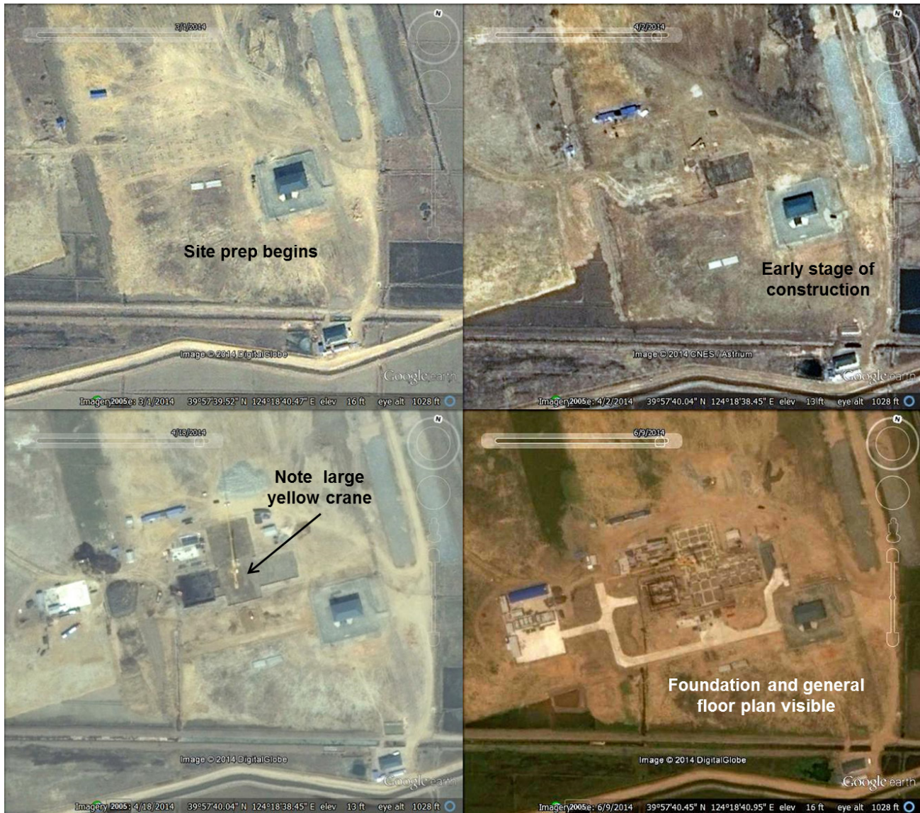
Figure 1. Construction on Hwanggumpyong begins early spring 2014.
