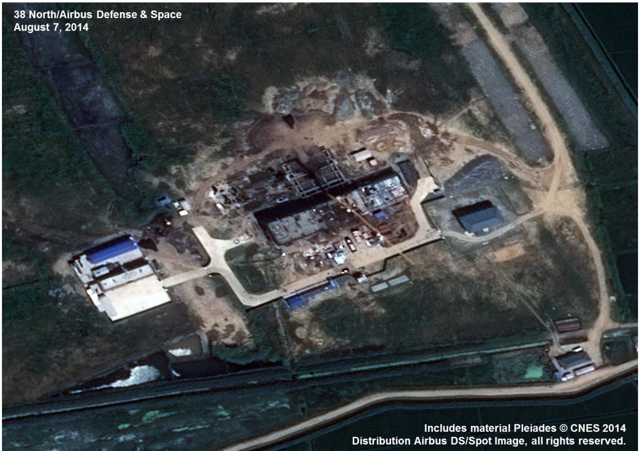
Figure 2. Significant progress made on building construction.
